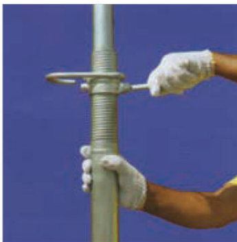
Set the pin into the hole of inner tube.
