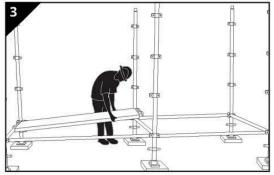
Fit the first working platform to ease the erection. Erect the complete working platform in the access bay.
