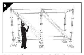
Fit the platform in each cell of the first stage. Stabilise the structure longitudinally by fitting diagonal braces at the side away from the working area (inset).
